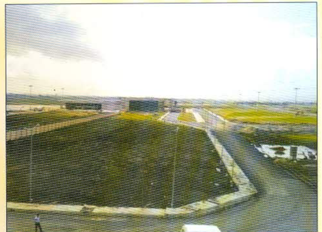
Land side aerial view of the airport.
